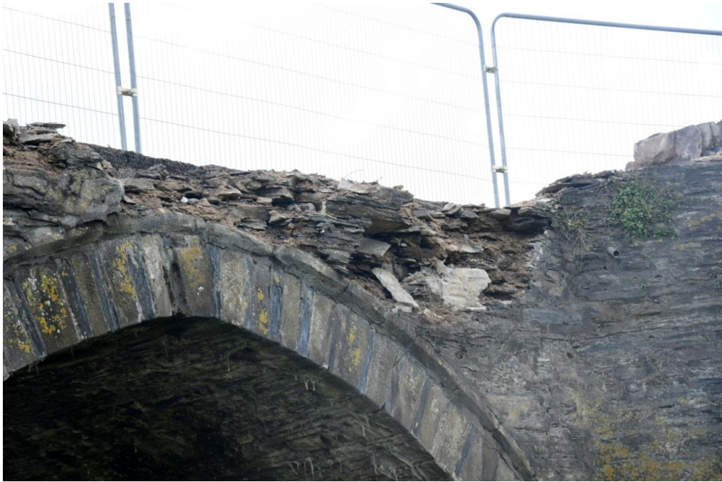
Damage to the spandrel wall as far as the voussoir
