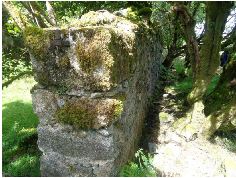
0.5m thick North wall showing metal gate hinge. Photo: Brian Oldham
