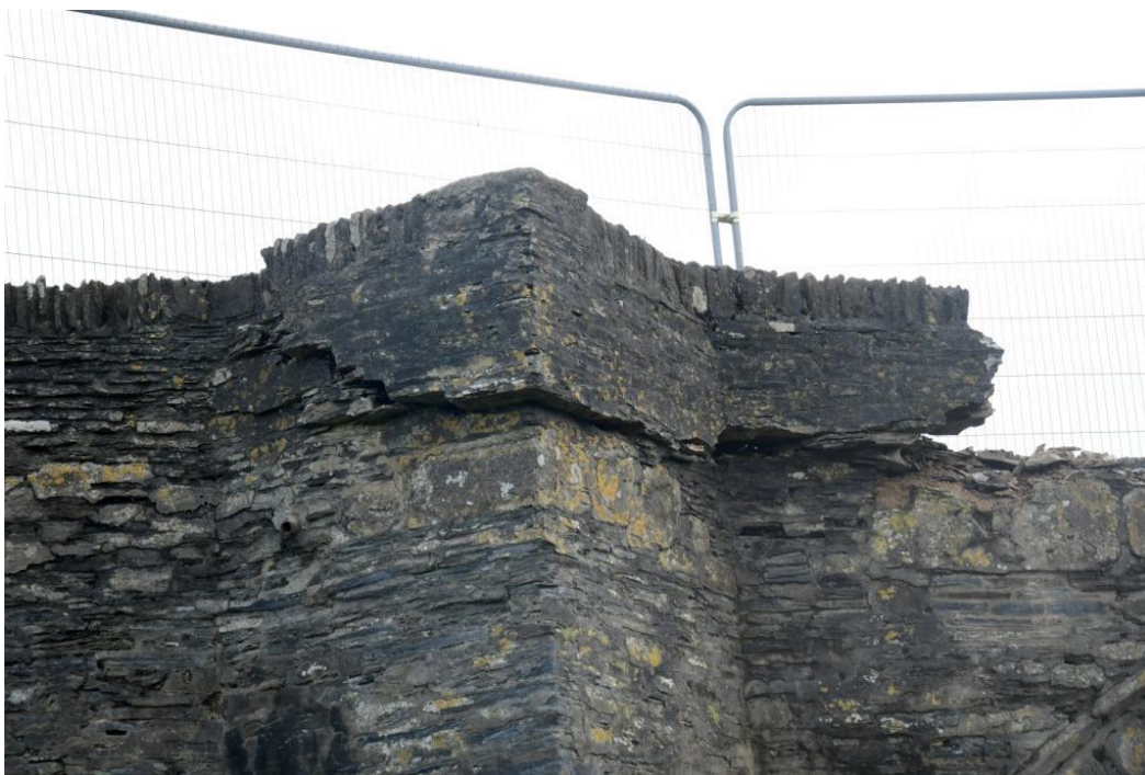
Wall of pedestrian refuge hanging over the edge of the bridge
