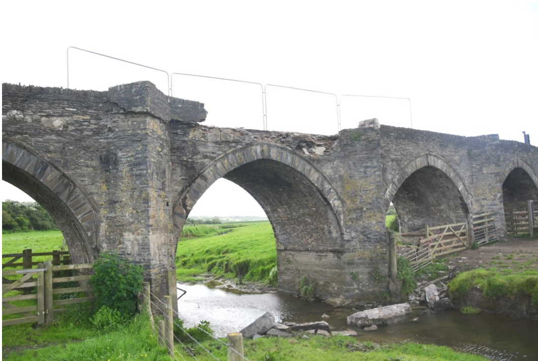
Upstream view of Trewornan Bridge showing large section of parapet missing
