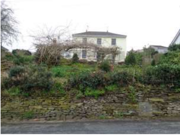
Grade II listed Wadeland House and front wall. jpg
